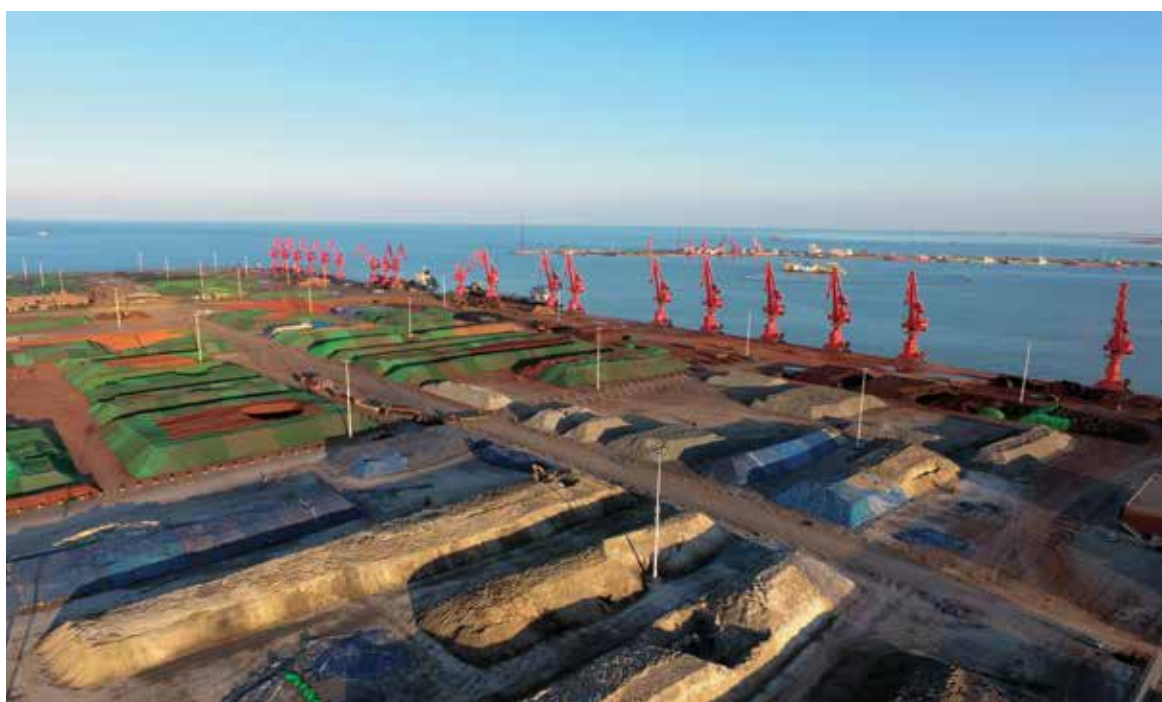
Dry Bulk Terminal at Weifang Sime Darby General Terminal Co. Ltd.
