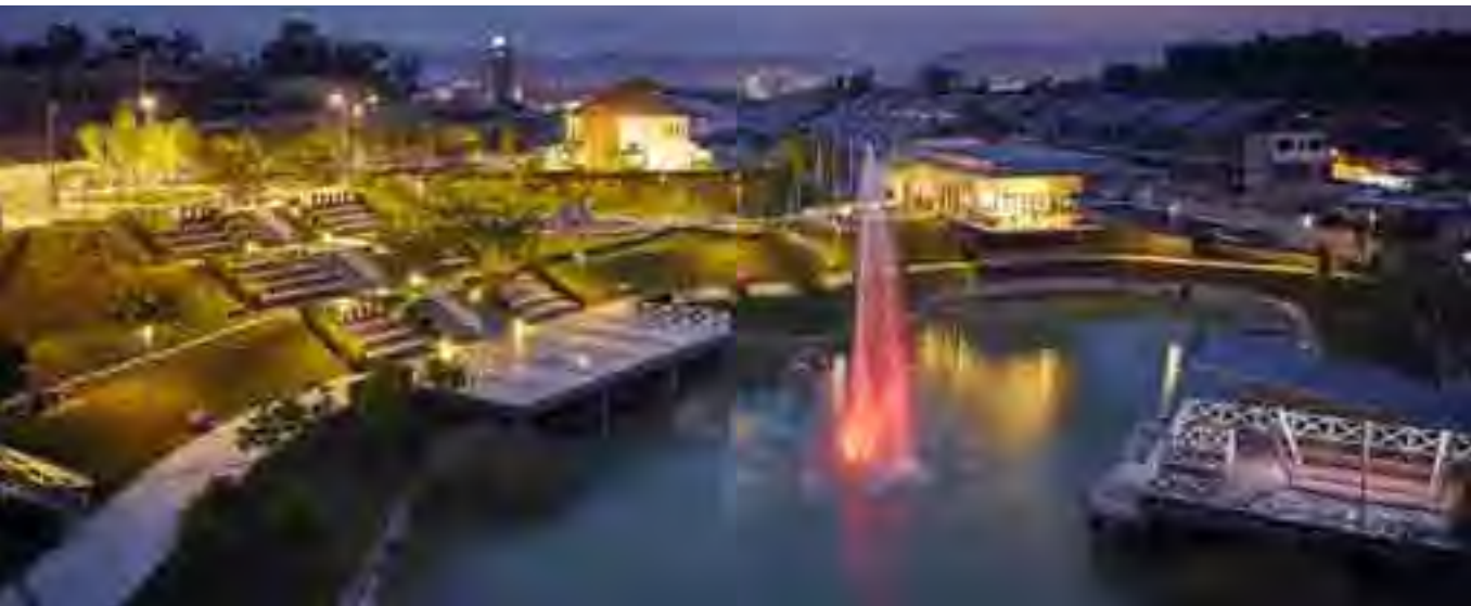
Chemara Hills, Seremban is a thoughtfully planned township nestled on elevated land, providing communities the space, privacy and security it needs.
