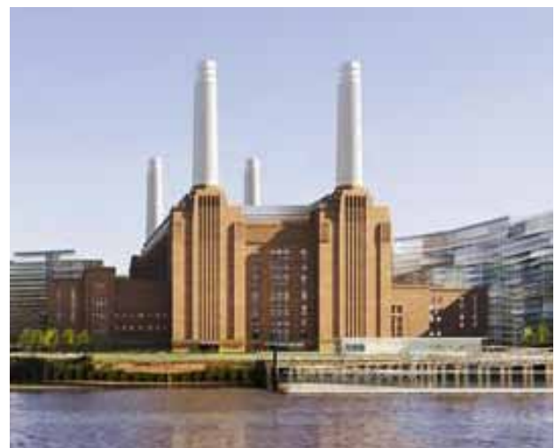
Battersea Power Station - a 39-acre mixed development in London, is a mega overseas project for Sime Darby Property
