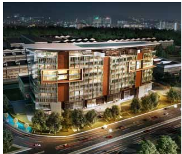
Artist's impression of the Melawati Corporate Centre – comprising office suites with F&B facilities and roof top terrace, with a magnificent view of the KLCC skyline and the Melawati Quartz Ridge
