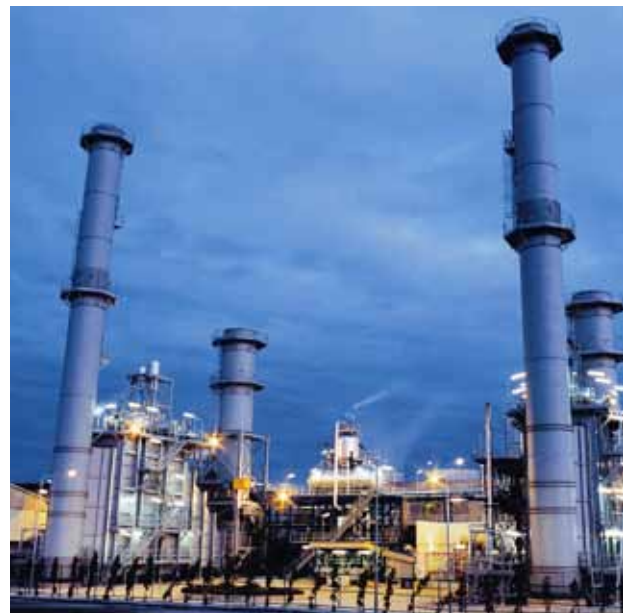
Night view of the Laem Chabang power generation facility. The power plants have a combined capacity of 180MW
