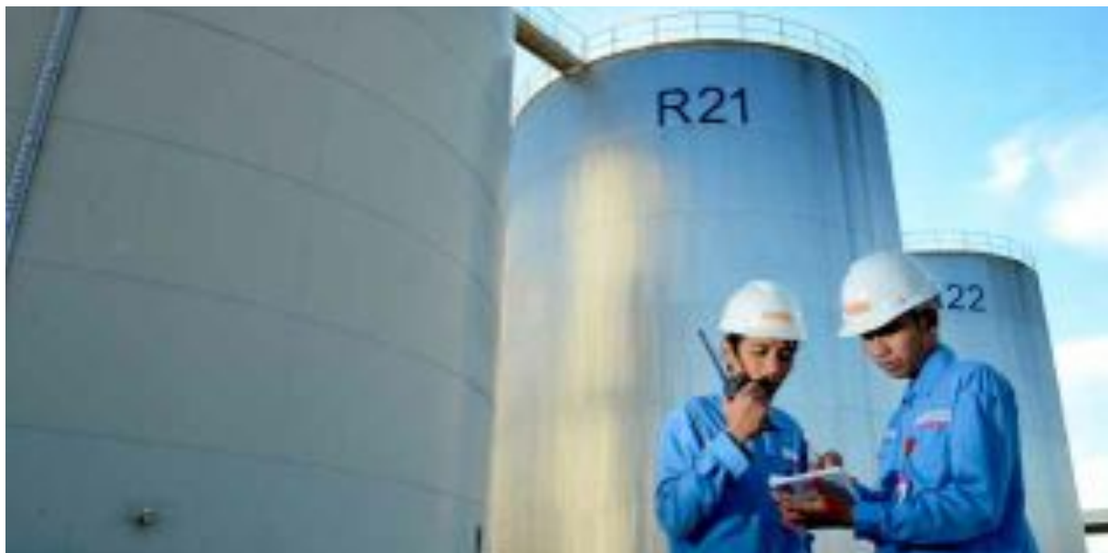
Efficient tank management is critical in optimising our Downstream's operations.
