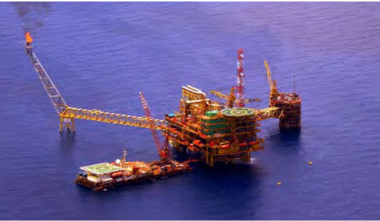
The expansion plan for the Oil & Gas business will strengthen the division's marine capabilities
