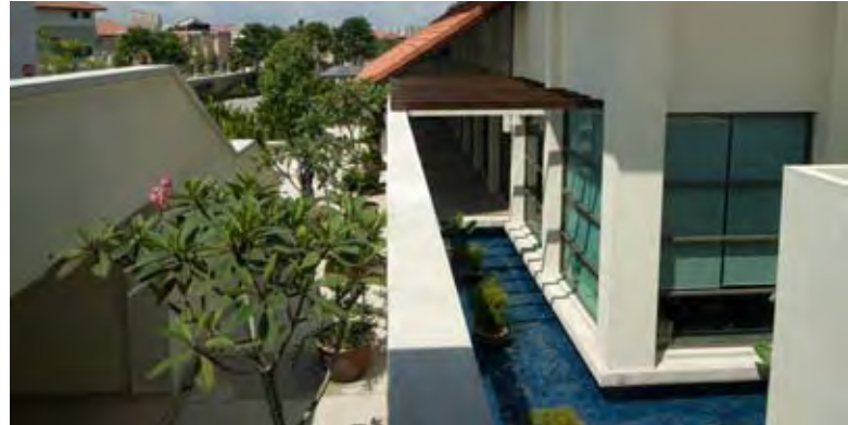
Phase 1 of the Ara Hill resort condominium is ready to be handed over in December 2009
