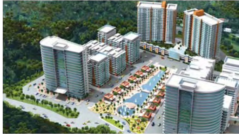
The Oasis project in Ara Damansara comprises commercial shop offices, retail outlets and serviced apartments
