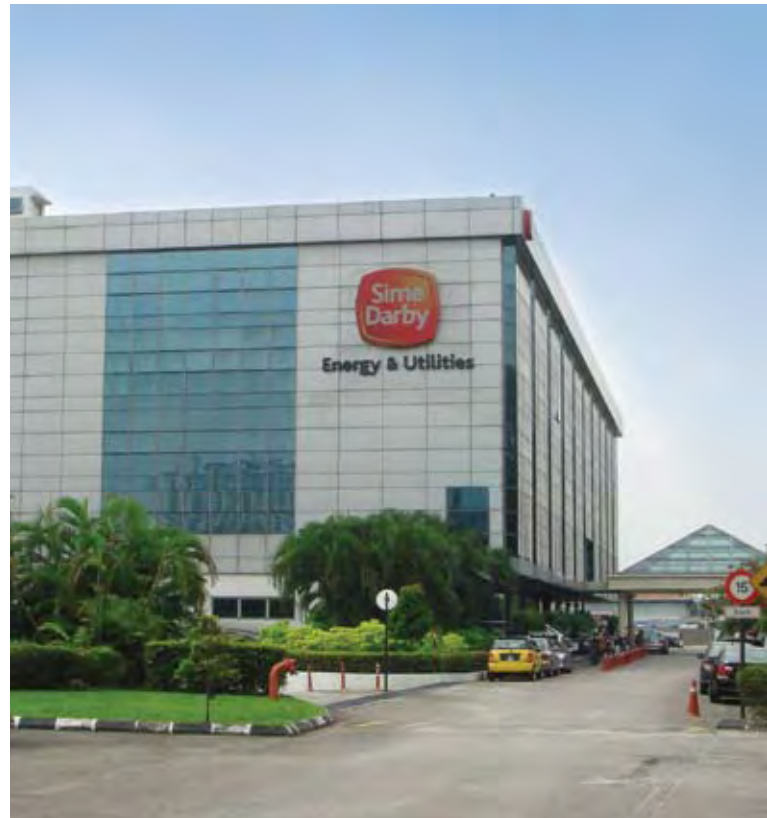
Various business transformation initiatives have been undertaken to turn around the Energy & Utilities Division
