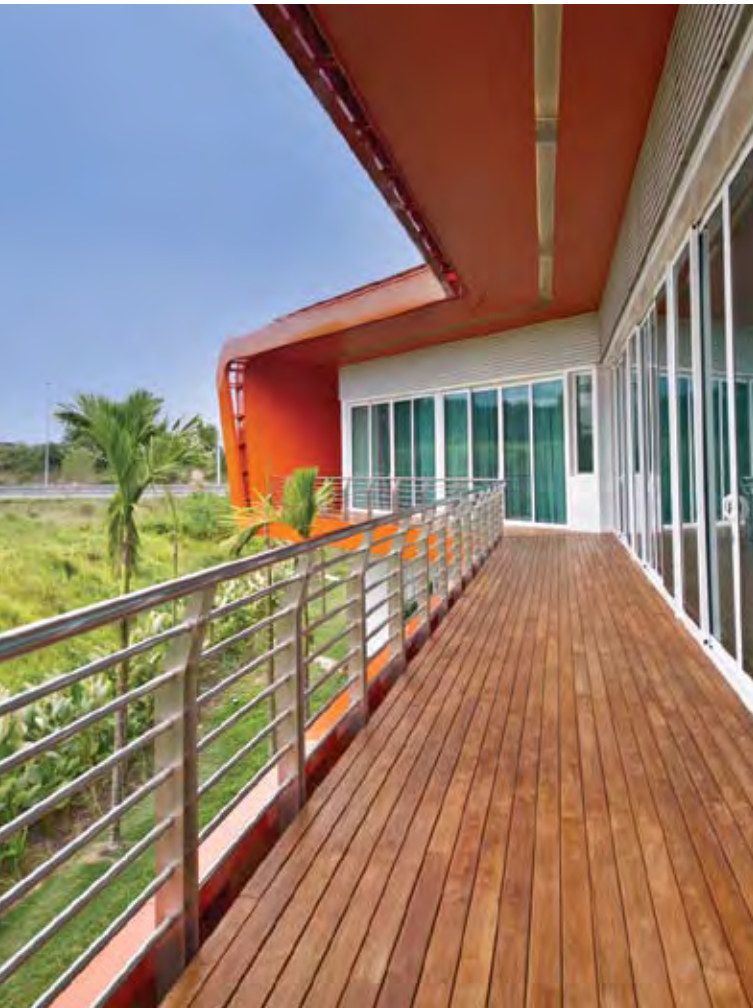
The Sime Darby Idea House in Denai Alam is a socially, economically, and environmentally responsive prototype dwelling that will provide an insight into future tropical living
