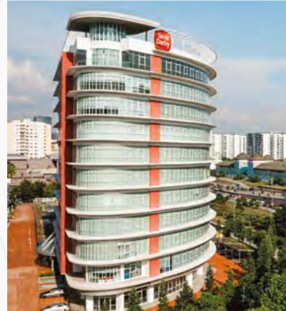
Sime Darby Berhad is headquartered in Menara Sime Darby, Selangor, Malaysia.
